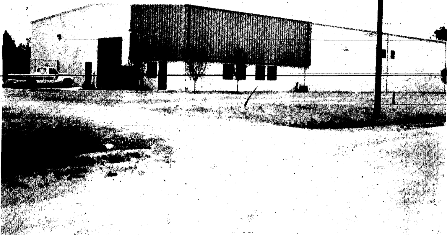
VILLAGE ELECTRIC AND WATER departments have moved to the new facility in the industrial park off Sibley Rd. Some final exterior work has to be completed and a large amount of dirt has to be removed. The former village building on North St. has contaminated soil and will probably have to be partially torn down as part of the clean-up process.
