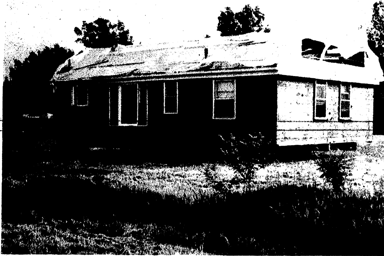
TEMPORARY RESTING PLACE for the former Van Buren St. home moved out of the village last Sunday is a field next to Vogel's Party Store on M-52 near Werkner Rd. Movers did not make all necessary arrangements for police escorts between Chelsea and Leslie, so the move had to stop at the village limits, which is as far as Chelsea police would go. There are several police jurisdictions between Chelsea and Leslie, northwest of Stockbridge.
